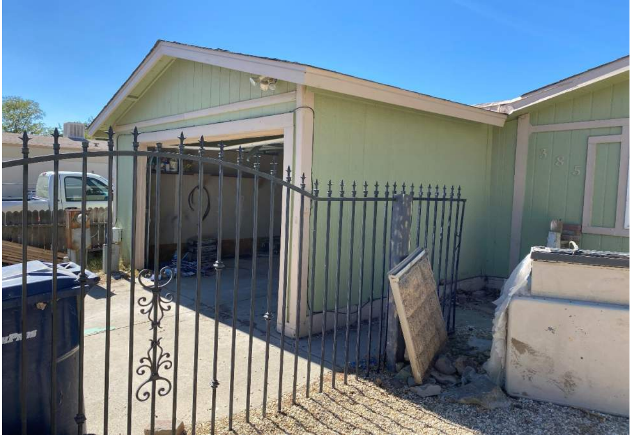
Looking southwesterly at existing attached garage (from Parkland Way)
