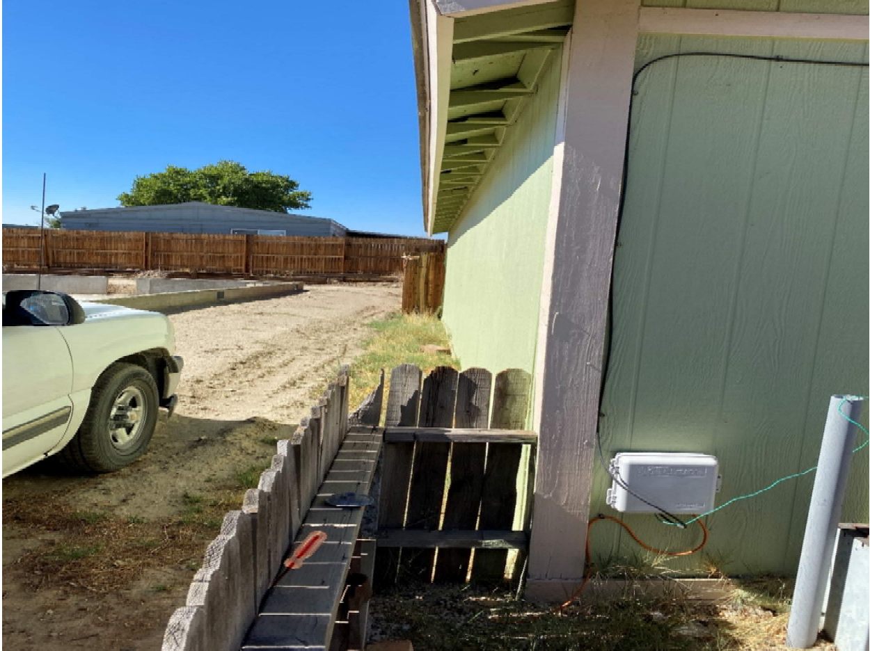
Looking westerly along south property line at garage proposed for zero lot line setback, with recently completed foundation on southerly adjacent 395 Parkland Avenue
